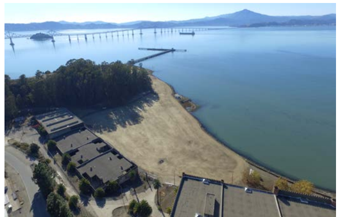
Clean closed site
