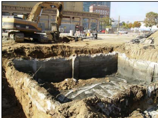
Sump removal during demolition.
