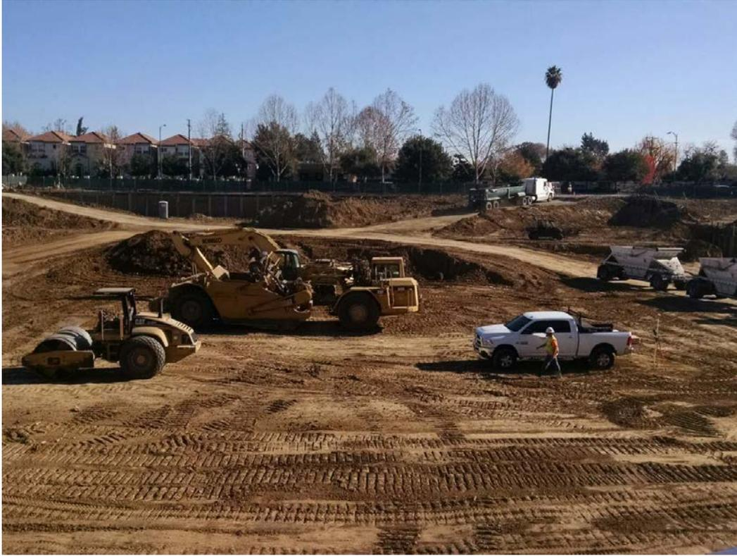
**DGC scraper and compactor support equipment in basement excavation area.**
