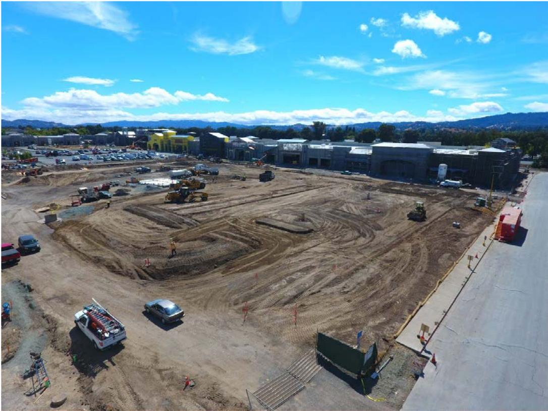
**DGC grading second phase of the parking lot while building construction is underway.**
